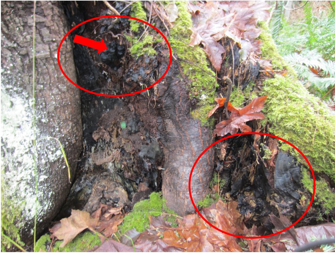
PHOTO 2: View of brittle cinder conk ( Kretzschmaria deusta ) on a bigleaf maple with basal damage. This is a dangerous tree and full tree removal is recommended. Cut with a high stump to remove the hazard while promoting coppice shoots for visual screening.
